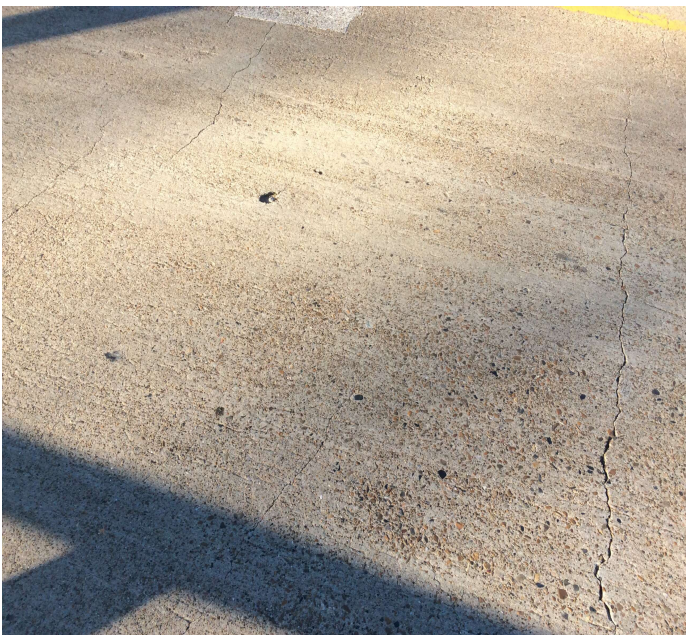
PHOTO 1 Description Deck cracks span 5
