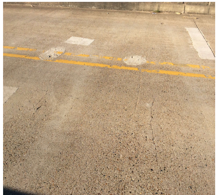
PHOTO 2 Description Span 3 deck cracks
